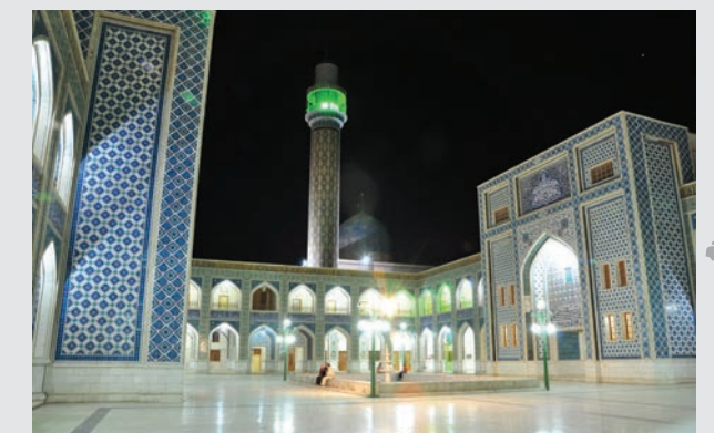
Shrine to Uwais Al-Qarani & Ammar Bin Yasser before damage/Photo: Wikimedia Commons.
