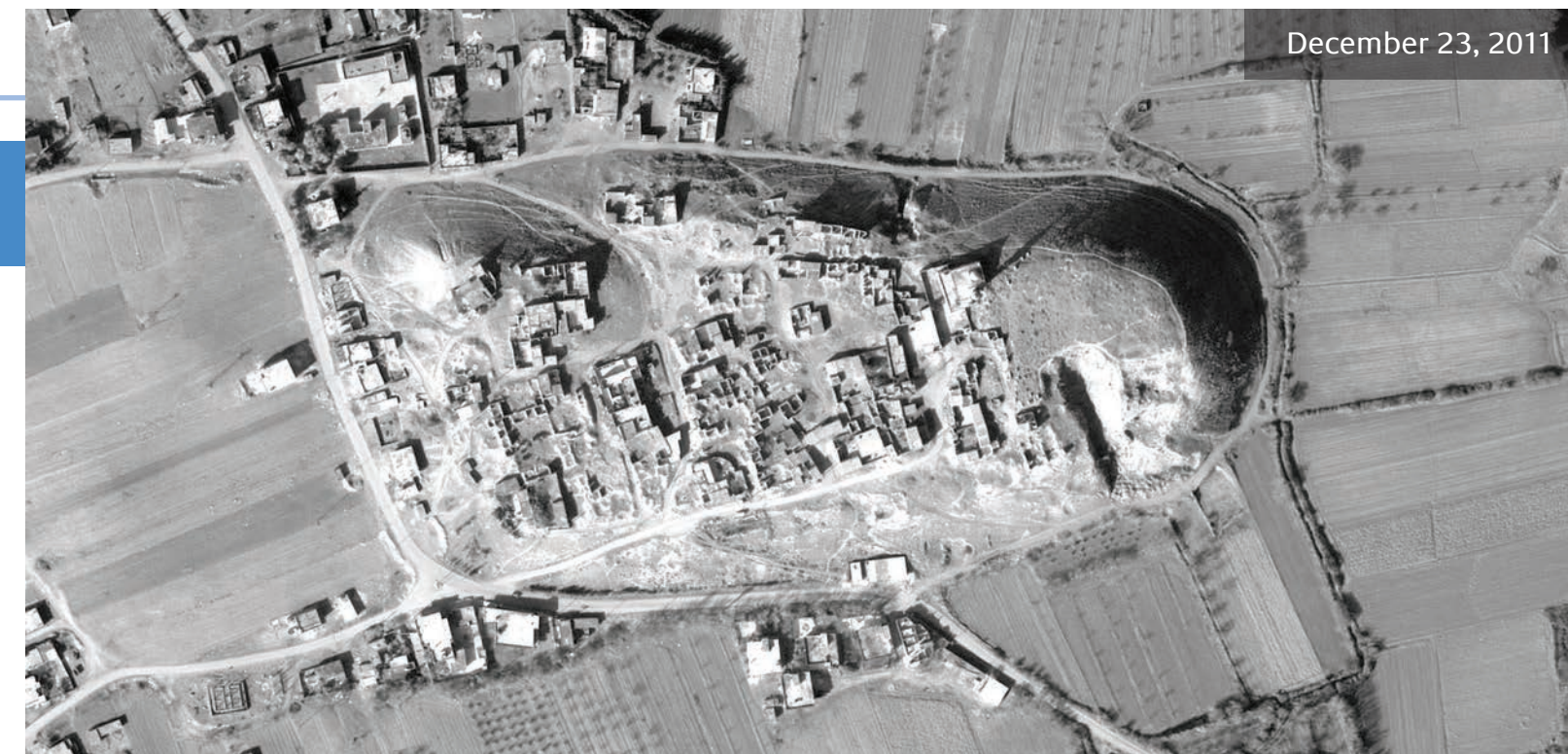
FIGURE 79. Qadesh before damage occurred.
