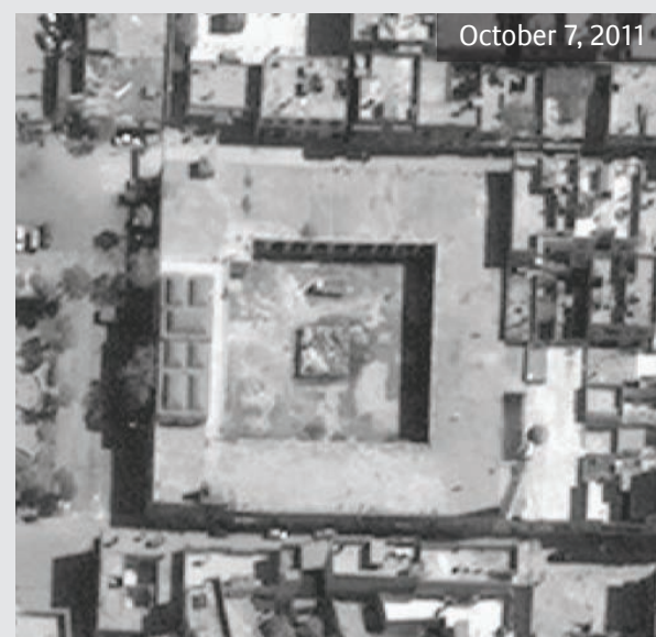
FIGURE 68. Damage to Khan Assad Pasha Al-Azem.
