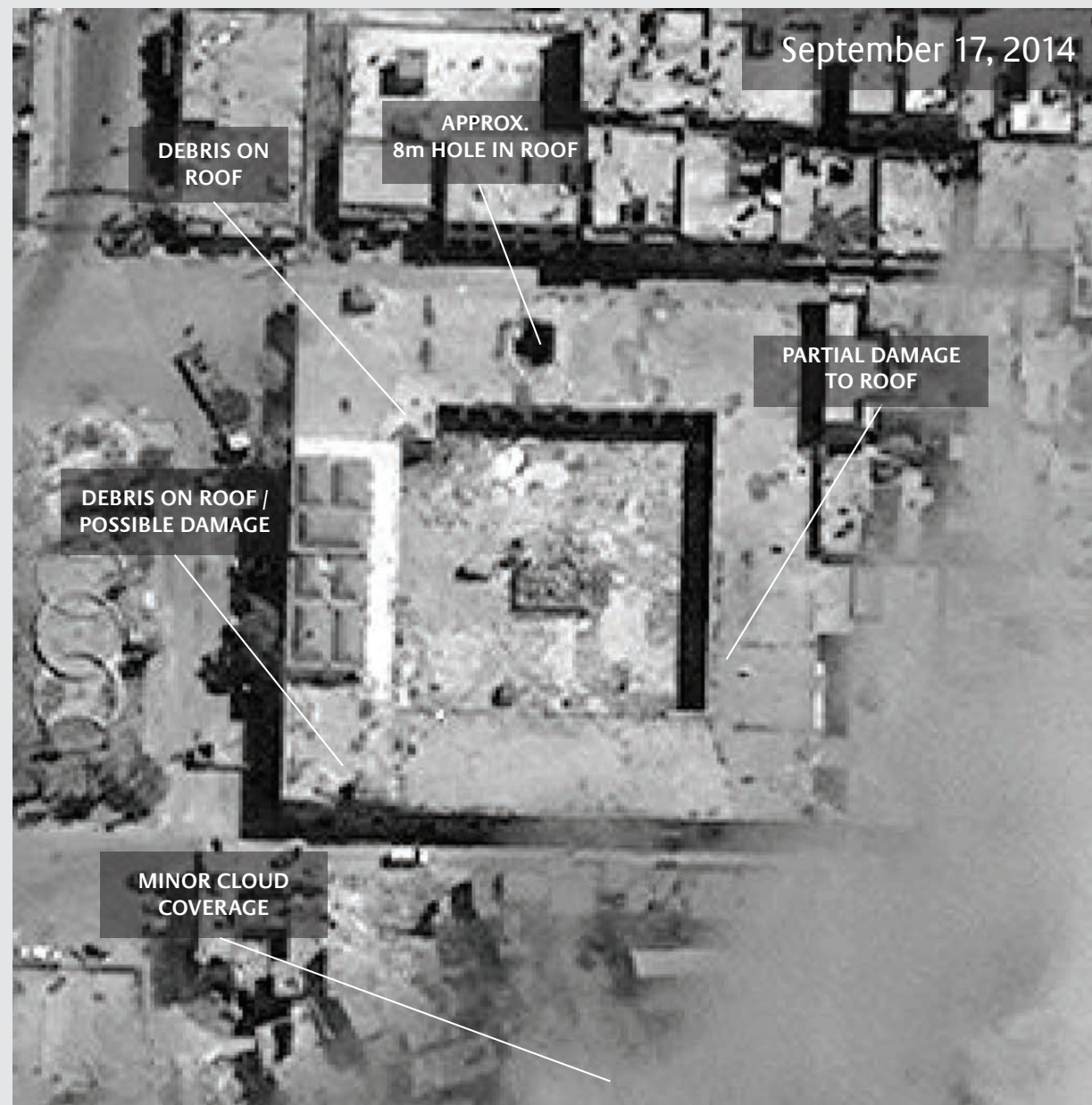
FIGURE 67. Damage to Khan Assad Pasha Al-Azem.
