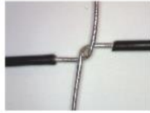
Figure 19-16. Initial Wrap for Western Union/Lineman Splice
