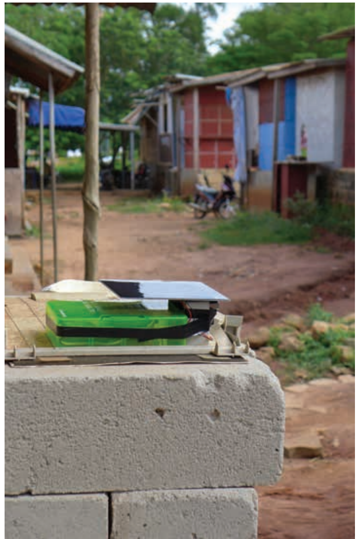
Photo credit: Marco Zennaro. Solar powered air quality sensor in Cotonou, Benin, sending data via SMS.
